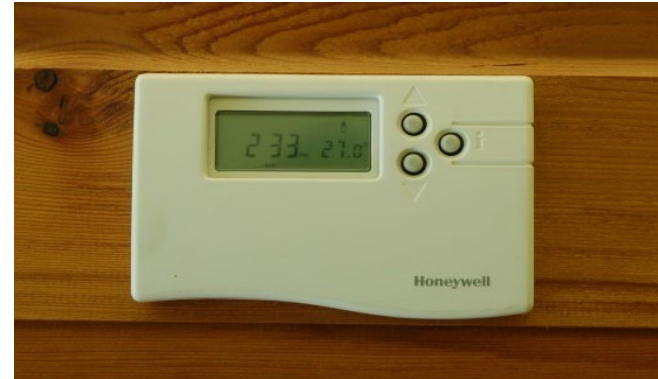
Thermostat in corridor set to 27°C in summer in Case Study C.
